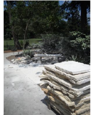
New flagstone waiting to be laid down on the southwest side.
